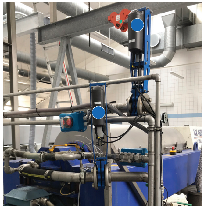
Pipeline with LINAK actuators. Dewatered sludge to anaerobic digester tank.
